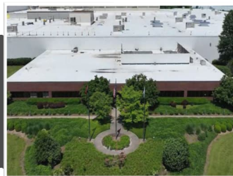
Clarksville, TN - advanced manufacturing facility
