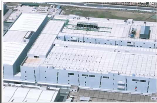
Cell, module, and pack building completed
