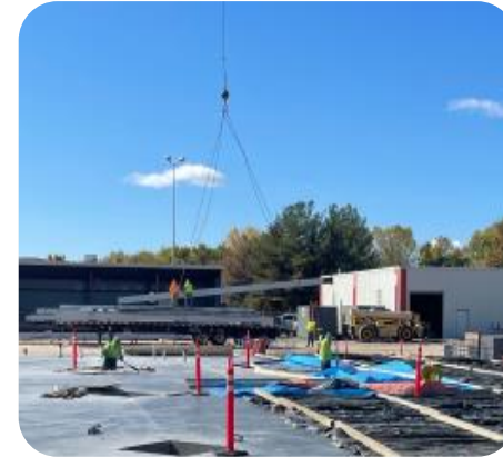
Clarksville plant under renovation estimated completion Q4 2023
