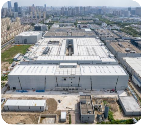
China Manufacturing Plant Expansion capacity expansion completed Q1 2023
