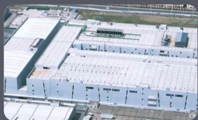
Cell, module and pack building completed
