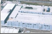
Cell, module, and pack building completed
